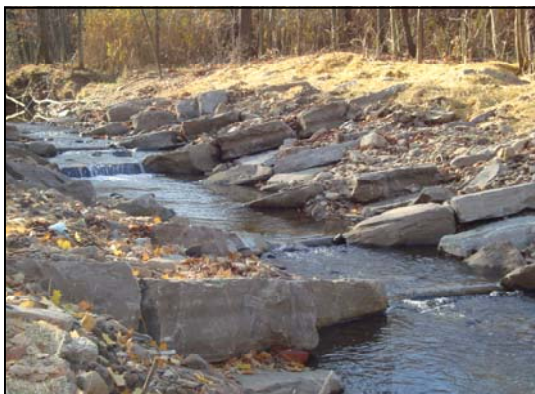
Restoration Site 11 (behind Midtown Towers, Broadview Road) Post Restoration - October 2010
